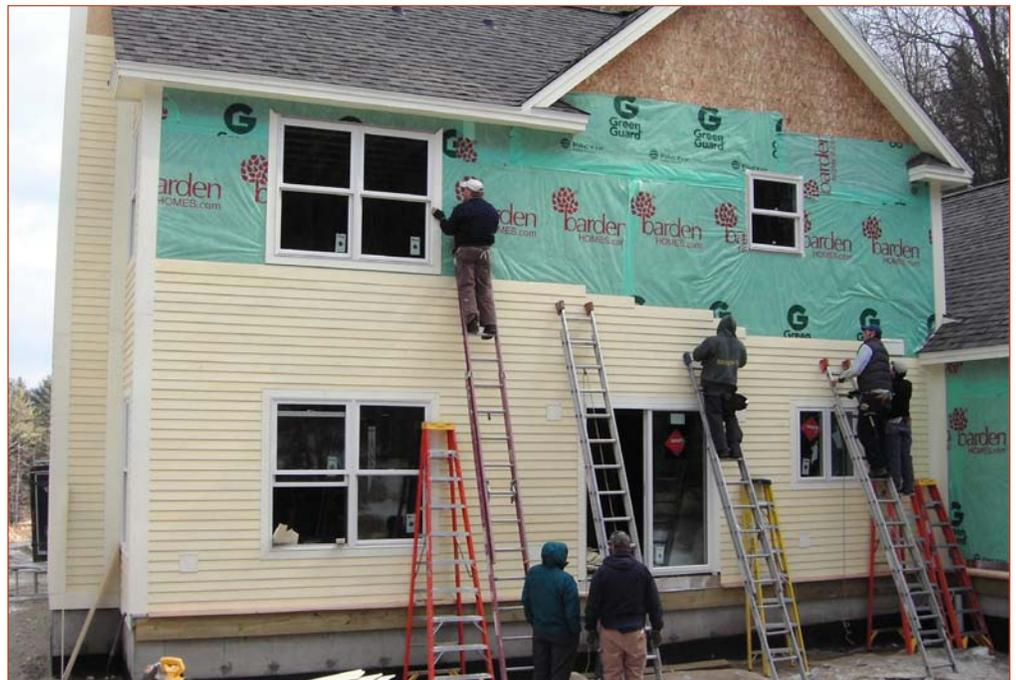
While some of the panels are still being set, other crew members get to work on other tasks, such as completing bridging and installing housewrap. Once the structure is complete, the entire crew can focus on windows, doors and siding.
