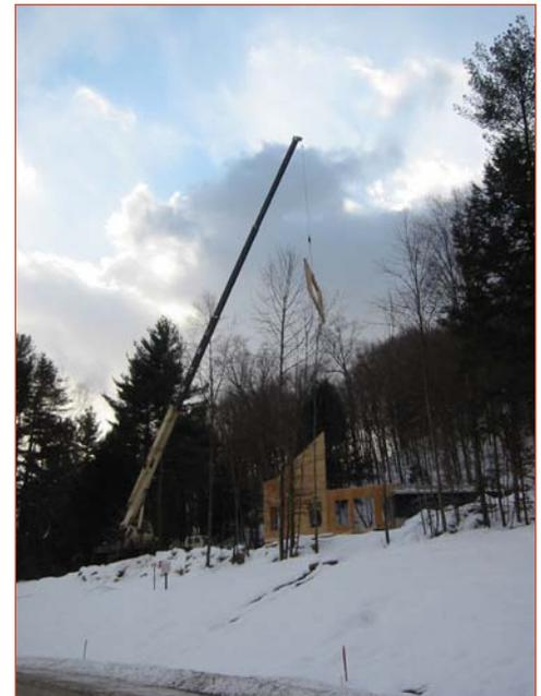
Vermont Built uses a six-man crew with a minimum of two men on the deck, one man on the truck hitching the chain, and one operating the crane. This allows the crew to set the walls for the first and second floors in two days.
