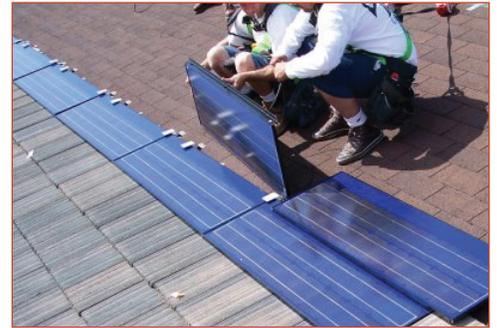
Carefully interconnecting each module, two crew members tie in the first two rows of the integrated PV system with the concrete roofing tiles.
