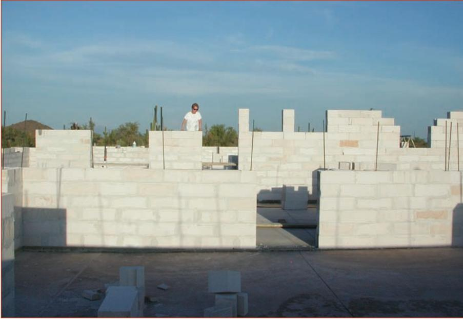
Steel rebar reinforces AAC block to create durable walls that easily meet load requirements.
