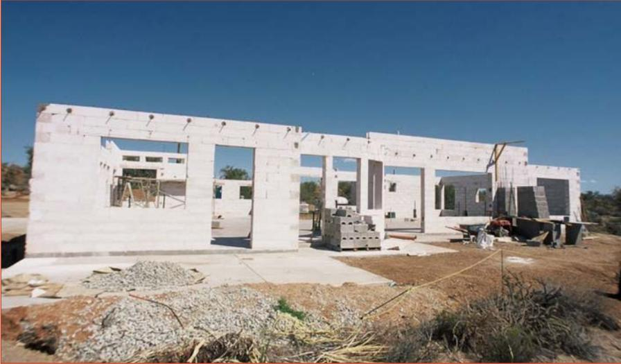
Walls built with AAC block are consistently straight, but can also be sculpted to meet a variety of architectural designs.
