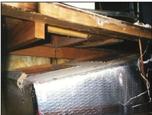
Completely disconnected air conditioning return plenum - easily avoided through independent inspection. (Florida Solar Energy Center photo)
