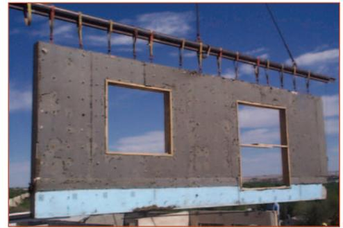
Extruded polystyrene (XPS) insulation, also referred to as blueboard, is placed at the base of the horizontal wall surface to create an FPSF.
