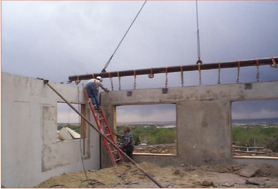
Field personnel work with the crane operator to line up the perimeter concrete walls. Horizontal insulation minimizes heat loss at building corners (see Fig. 1).
