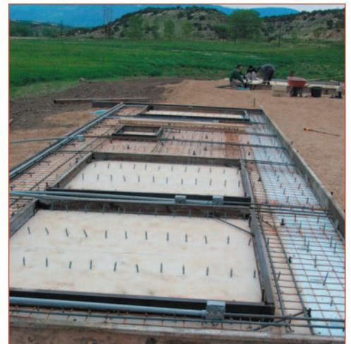
Prior to tilt-up, cast-in-place concrete walls are fitted with 2” extruded polystyrene (XPS) insulation, electrical boxes, and blockouts for windows and doors.
