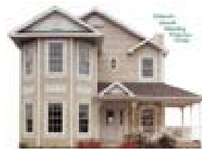
Victorian house constructed with a hybrid modular and panelized approach Source: ToolBase Website ( www.toolbase.org )
