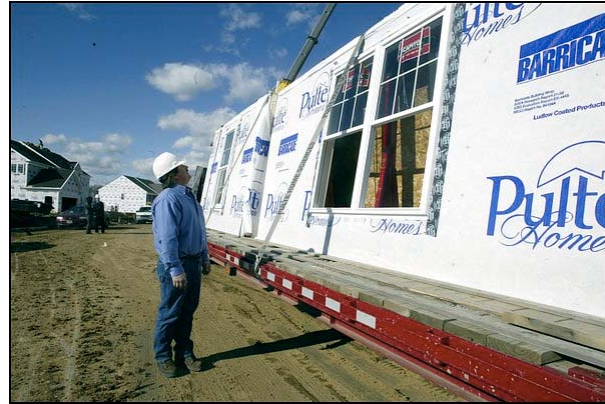
Prefabricated wall panel being set on a site Source: Washington Post, Photo by James A. Parcell
