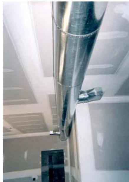
A minimized duct layout at a PATH field evaluation site. The duct system utilizes short supply takeoffs and is located within conditioned space.
