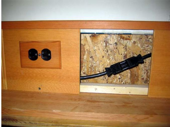
Modular connector for pre-wired wall panels
