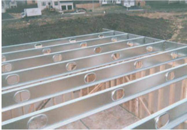
Dietrich TradeReady® joists spaced at 32" O.C. To accommodate this wide spacing, 1-1/8" thick floor sheathing was applied.
