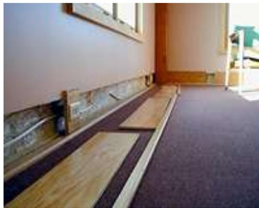
Prefabricated wiring chases in Bensonwood's factory-built walls
