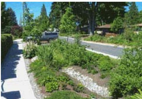
▣ Figure 3: Example of a Swale
