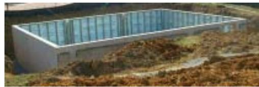
Precast wall panel by Superior Walls from PATH Field evaluation
