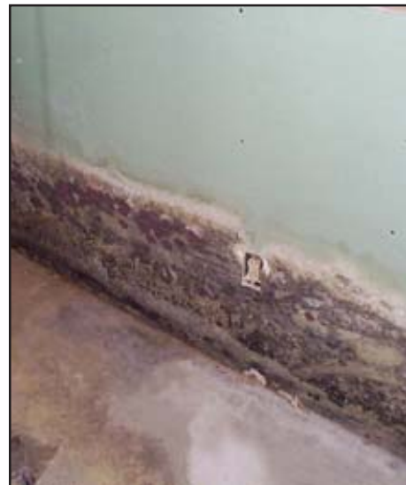
Courtesy: Steven Winter Associates, Inc.
