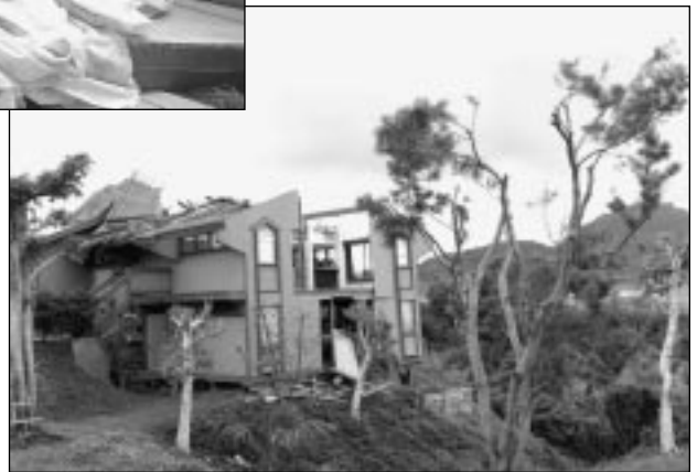
Hawaii, September 1, 1992 -- The roof and upper floor of this home received major wind damage from Hurricane Iniki.
