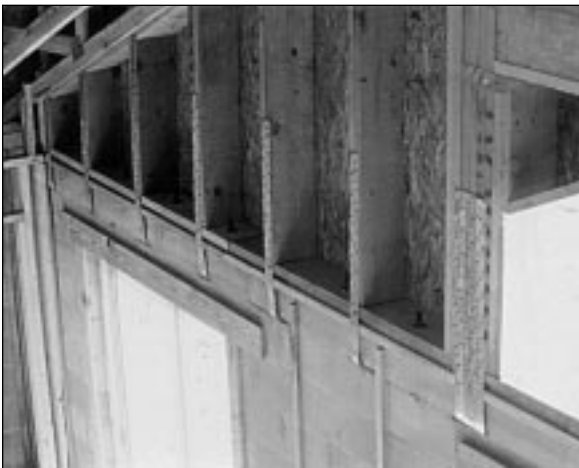
Southport, NC. FEMA mitigation specialists Sharon Steen and Diane Earl inspect the hurricane straps that were added to this home. The straps provide additional protection to the home during high winds. Photo By Dave Saville/FEMA News Photo
