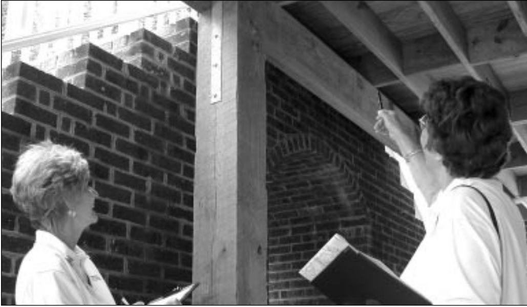
Southport, NC. FEMA mitigation specialists Sharon Steen and Diane Earl inspect the hurricane straps that were added to this home. The straps provide additional protection to the home during high winds. Photo By Dave Saville/FEMA News Photo
