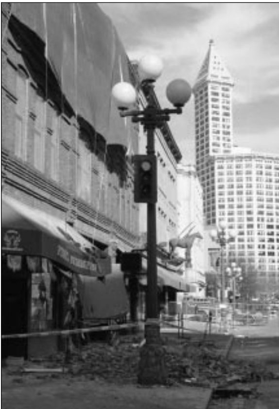
Seattle, WA, March 5, 2001 -- There is substantial earthquake damage in Pioneer Square, part of Seattle's historic district. Photo by Liz Roll/FEMA News Photo
