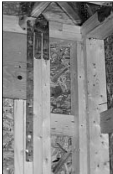
Southport, NC. FEMA mitigation specialists Sharon Steen and Diane Earl inspect the hurricane straps that were added to this home. The straps provide additional protection to the home during high winds. Photo By Dave Saville/FEMA News Photo
