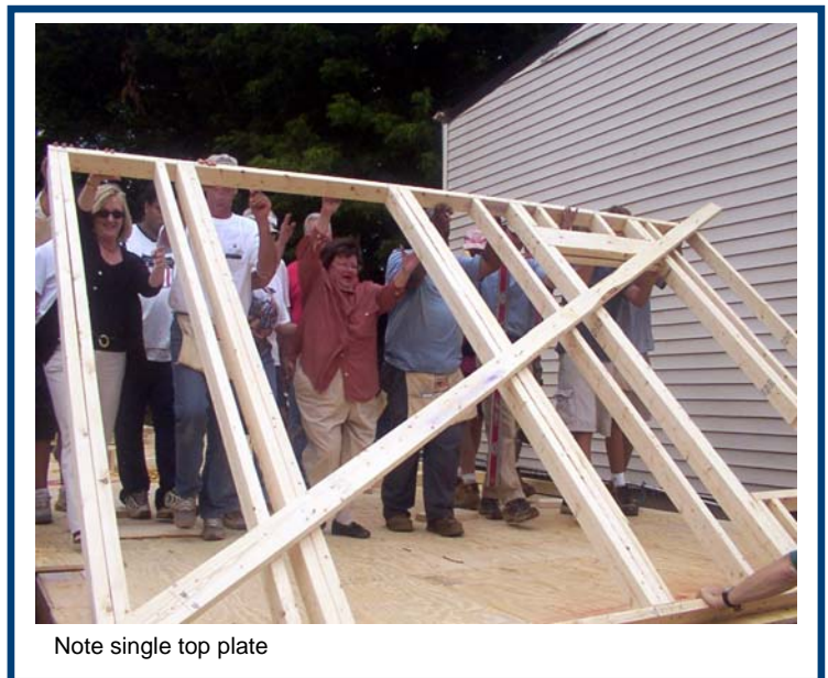
Figure 1 - The first wall is raised
