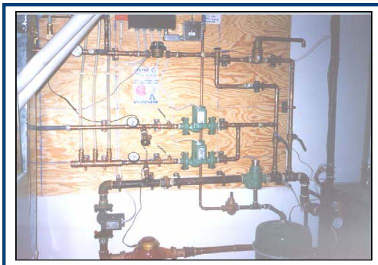
**Figure 3 Radiant system piping layout
