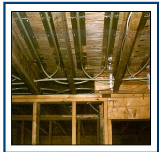
**Figure 3 Supply and return manifolds for the second floor (zone valves located on the upper manifolds)**
