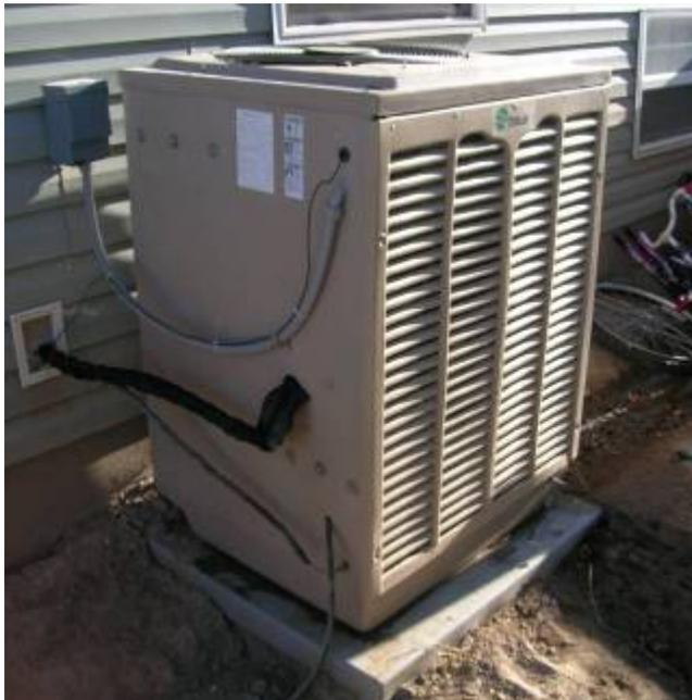
**Figure 2. Freus Evaporative Condenser (Unit A)**
