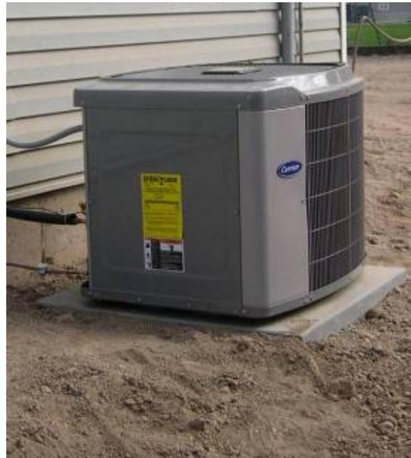
**Figure 3. Air Cooled Condenser (Unit B)**
