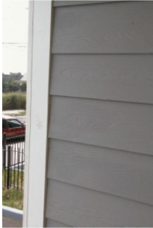
Fiber cement siding at Springfield Village
