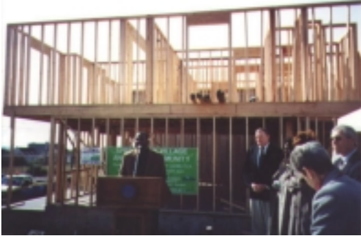
Construction site open house at a two-family model
