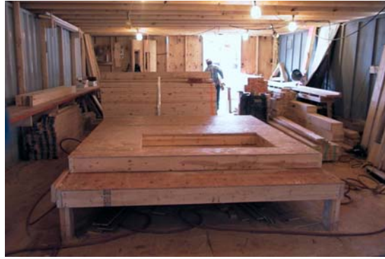
Wall panels assembled in temporary on-site construction “shack”
