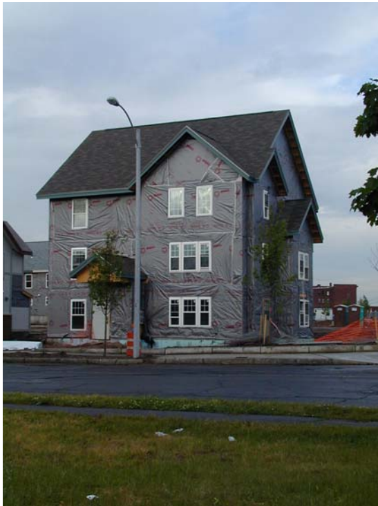
Three-family house during construction
