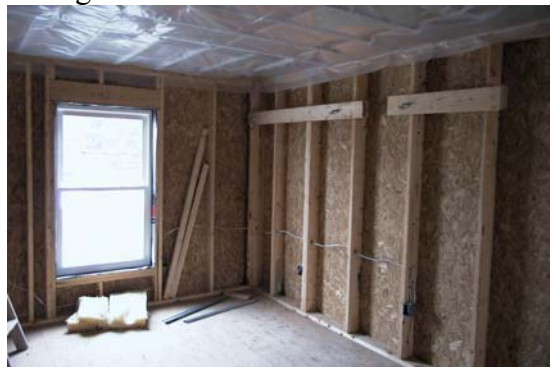
Wall framing studs at 24 in. on-center
