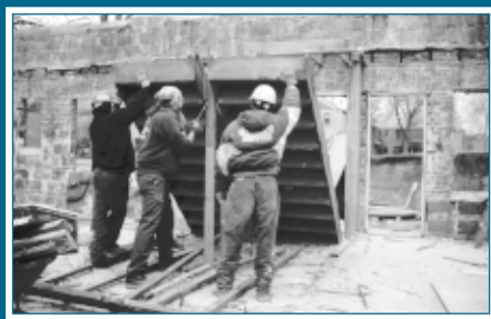
Stair removal – Riverdale Village.
