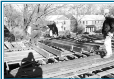
Floor system disassembly.
