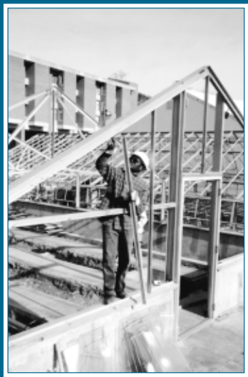
Greenhouse frame assembly— Walter Reed Army Hospital.
