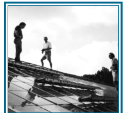
Building assessment – Walter Reed Army Hospital.
