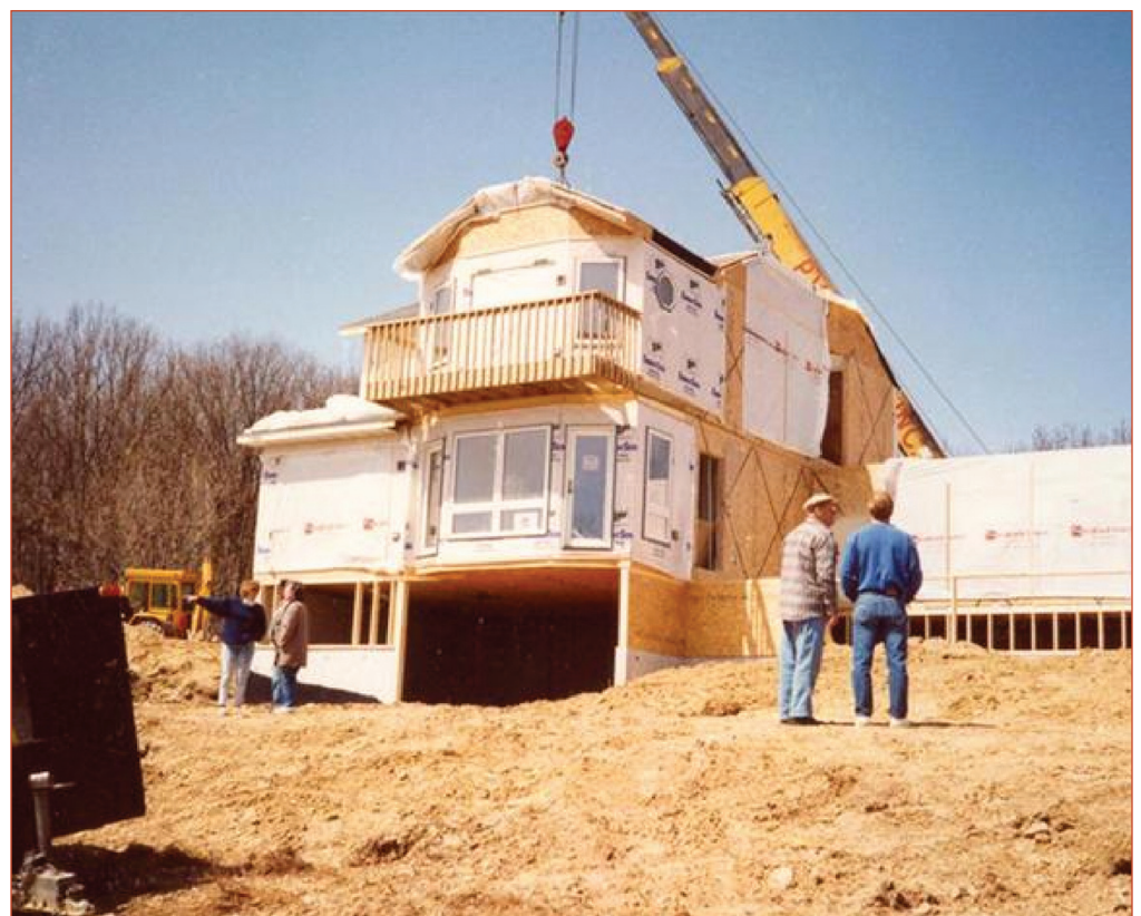
A crane carefully lowers a module into place.
